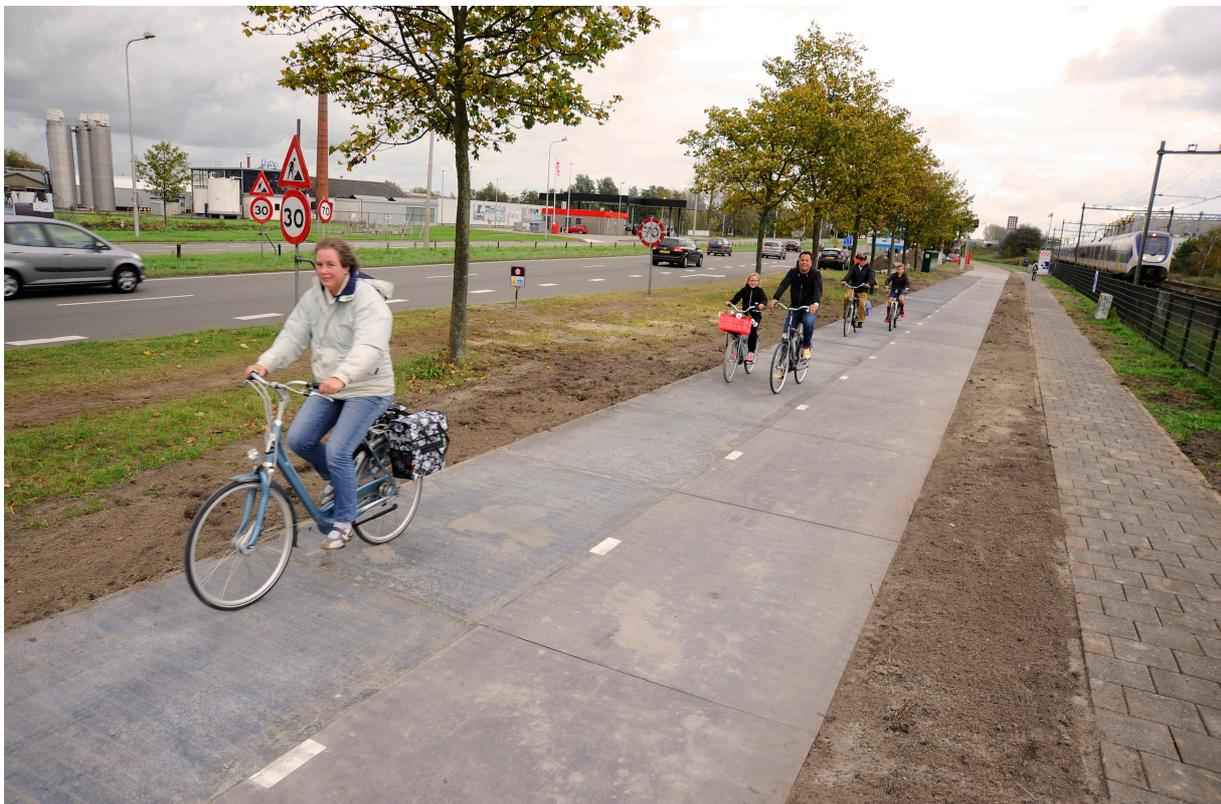
**The SolaRoad pilot road has been opened this week. SolaRoad is a road surface that acts as a solar panel. SolaRoad will be officially opened on the 12<sup>th</sup> of November by Minister Kamp. This is the first road in the world that converts sunlight into electricity. SolaRoad was developed by TNO, the Province of North-Holland, Ooms Civiel and Imtech Traffic&Infra.**
